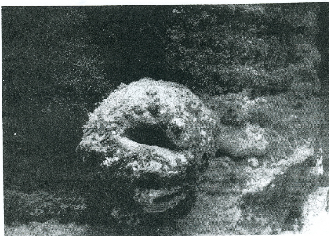
Fig. 12. Detail of artificial Reef 1 after accretion.
